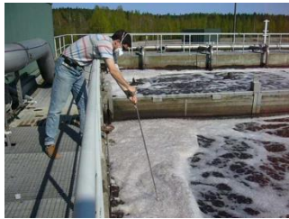
Waste water treatment plant
