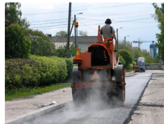
Asphalt paving machine
